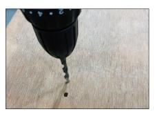
+ Drill six 7mm holes for the Tee Nuts.
